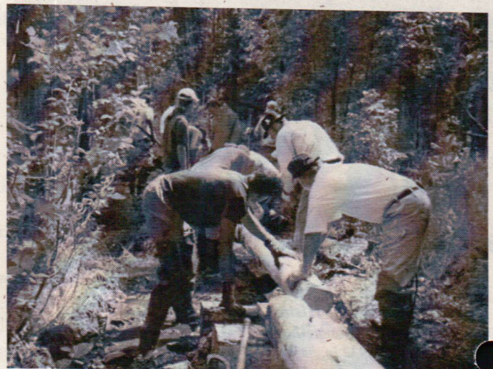
FENW volunteers making a log bridge over a wet area on Meadow Creek.
