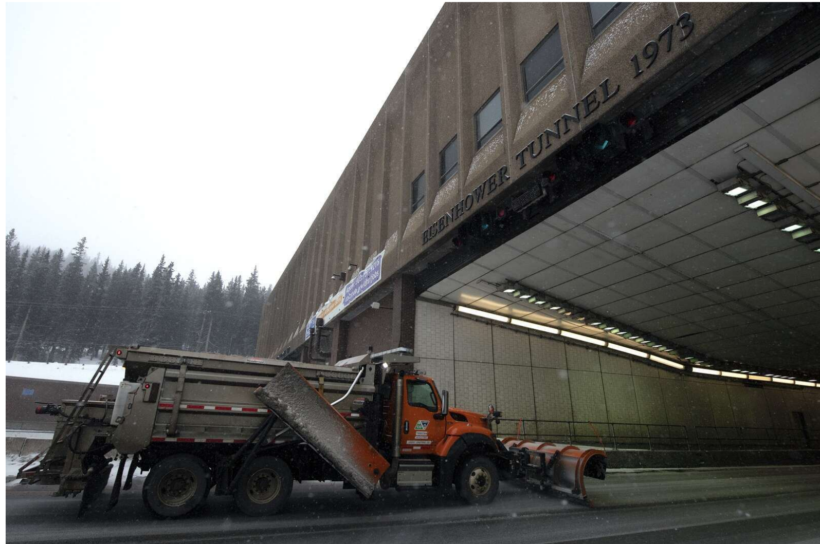
A Colorado Department of Transportation plow truck drives toward the entrance of the Eisenhower Tunnel during the start of a snowstorm Feb. 1.
